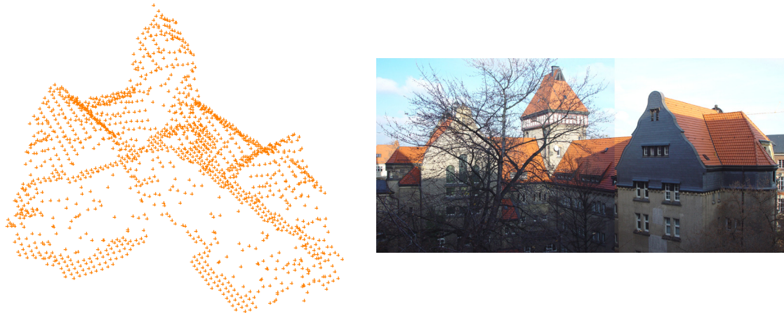
Figure 3-27: Point cloud and picture of the Tillich-Bau of the Dresden University of Technology
