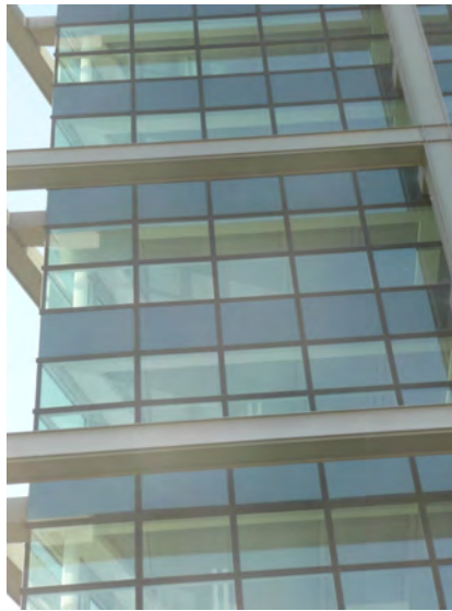
Fig. 48. Structure of the main railway station, Berlin. Left: Horizontal and vertical bars surrounding the building. Center: The facade is made of glass and partly covers concrete separating different floors of the building. Glassy surfaces are connected by metallic structures. Right: Corners occurring at the intersection area between horizontal and vertical bars. For all floors of the building, these corners can be found on the front and back side of the vertical bars. Corner sidelength: approx. 5 cm.
