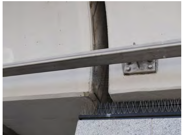
(b) Constructional gap at bridge that allows for different motion directions of bridge segments, i.e., observed movement towards each other during summer times.
