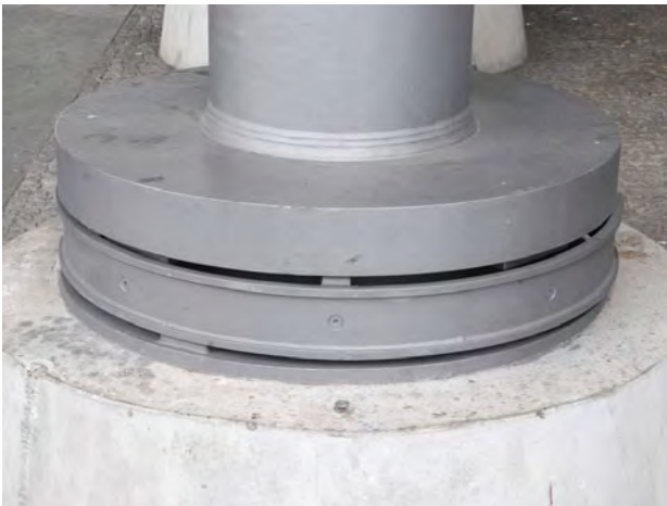
(a) Special mounting of piles enabling horizontal movement in any direction.
