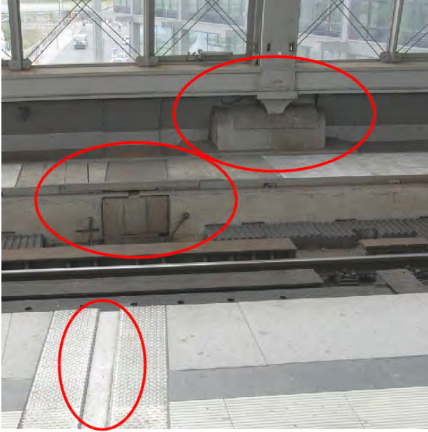
(a) Three special constructions, enabling horizontal movement for the halls and both sides of the station platform. Locations highlighted by red ellipses.
