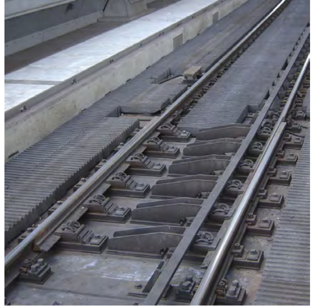
(b) View on the separation of the rail tracks. The detached parts along direction of train allow for large horizontal movements.
