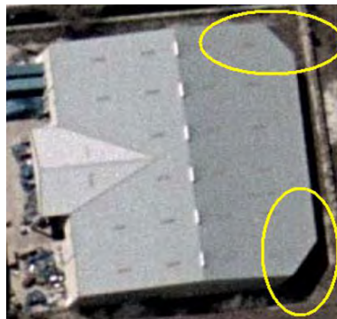
Figure 1.7: Insignificant irregular edges within the building outline (yellow color ellipse).
