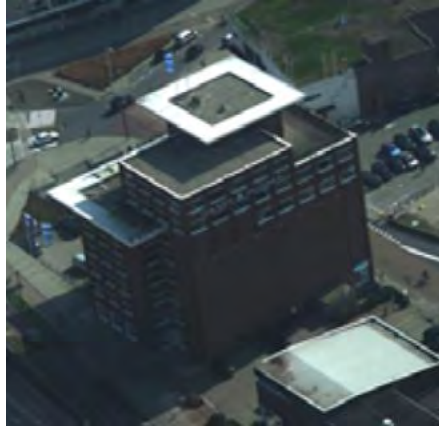
Figure 1.2: Oblique image of a high-rise building with polygonal height jumps (Oude Elberink, 2010).
