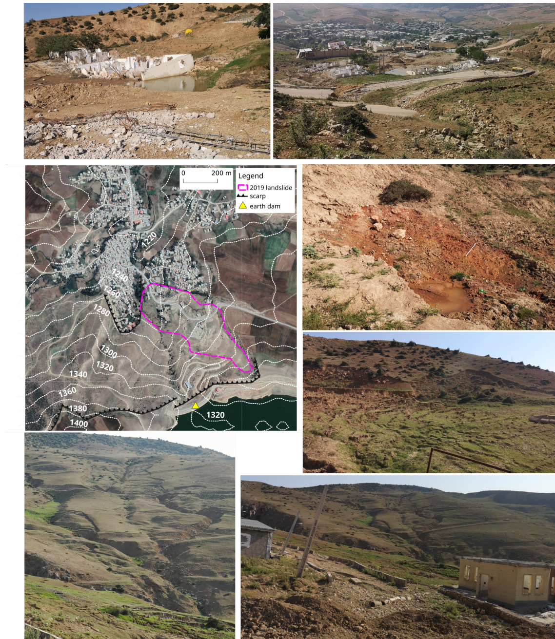
Figure 5.2: Field photos of the landslide area from July 2019: (a) damaged buildings and sag ponds; (b) damaged road on the upper part of the landslide; (c) post-failure satellite optical images over Hoseynabad-e Kalpush village from June 2019 (Google ©Imagery CNES/ Airbus Maxar Technologies) same extent as red rectangle in Fig. 5.1a; topographic contours (white lines) derived from the 30 m resolution Shuttle Radar Topography Mission (SRTM) digital elevation model; yellow rectangle locate the dam; magenta outline shows the landslide extent; (d) sag ponds in proximity to the north-eastern flank; (e) tension cracks and fissures on the landslide northeastern scarp (f) and (g) Southwestern adjacent old landslide showing gully erosion features.
