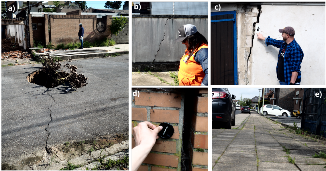
Figure 3.1: Fieldwork photos depicting building and infrastructure damages due to land subsidence: a and b from Maceio’ (Brazil) taken in December 2022; c , d and e from Hambach area (Germany) taken by M. Vassileva in June 2023
