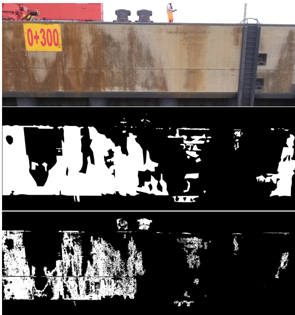
Figure 1. Example of a cropped RGB image showing the east-facing sheet pile wall of the JadeWeserPort and corresponding weakly and manually supervised ground truth images (top to bottom).
