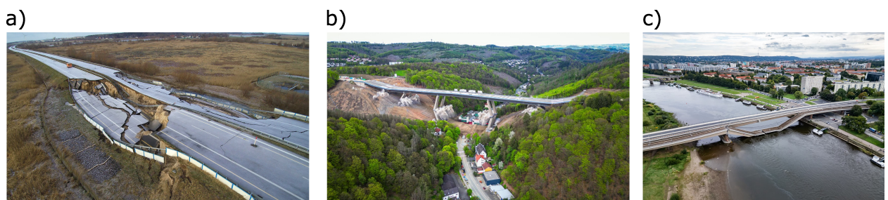
Figure 1.1: Examples of vulnerable transport infrastructure in Germany. a) Subsidence at the A20, Tribsees (Photo ©Stefan Tretropp). b) Demolition of the Rahmedetal-bridge, Lüdenscheid (Photo ©Daniel Schröder). c) Partial collapse of the Carola-bridge in Dresden (Photo ©picture alliance/dpa, Robert Michael).
